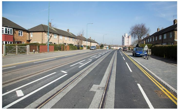
This contract involved the supply and lay of 80,000 tonnes of asphalt and laying cement bound materials (CBM) on highways, car parks, footpaths and between the tram tracks as phase 2 of the NET network was constructed across Nottinghamshire.
