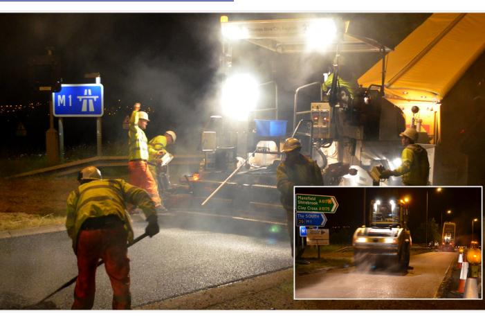
Working on behalf of Derbyshire County Council, these works formed part of our Surface Work for Highways Framework Contract. Working nights, our task was to resurface two major roundabouts to the M1 J29 and J30 using a 10mm Polymer Modified Binder (PMB) surface material, and road studs and road marking to complete.
